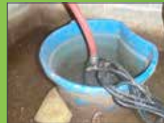
DAMAGED SUMP PUMP
